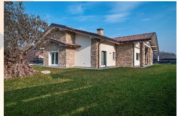
Small Villas Heating
